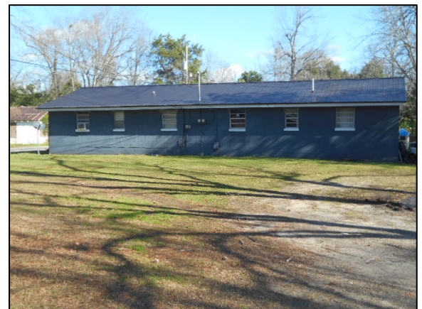
Single-family detached home north of site.
