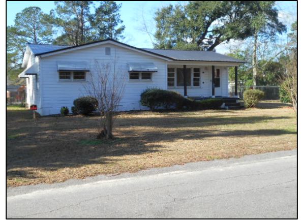
Single-family detached home west of site.
